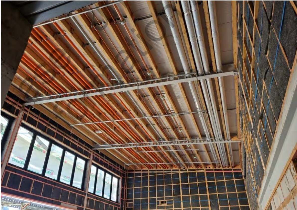
10207 – Acute Mental Health and Addictions Facility (Te Whare Awhiora), Tairāwhiti Services reticulated through ceiling
