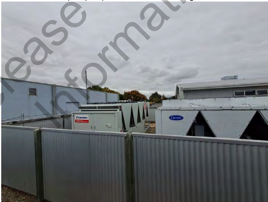
New chiller-heat pump in position next to existing chillers
