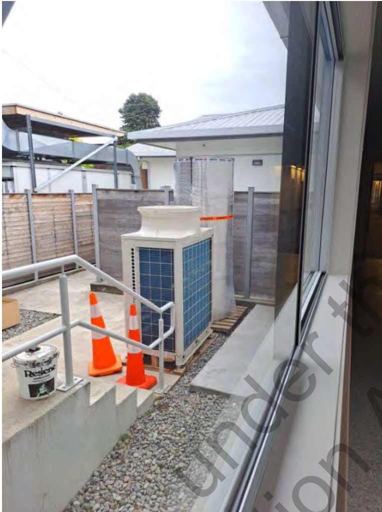
New chiller-heat pump in position next to existing chillers
