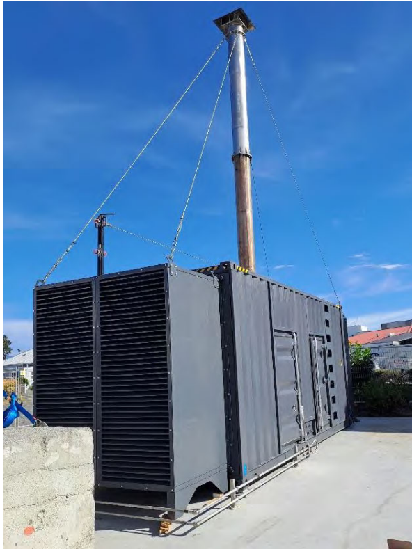
First generator on site
