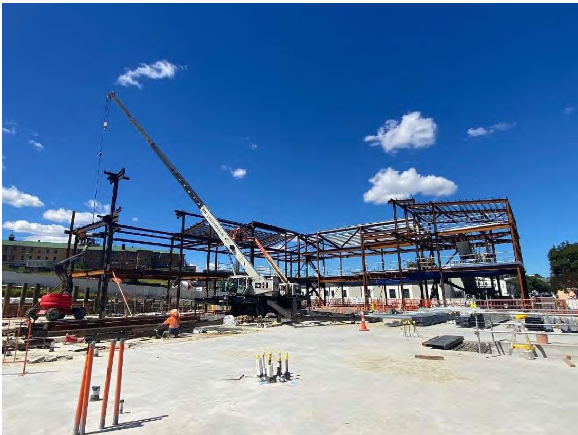
Structural steelwork in Zones 2 and 3
