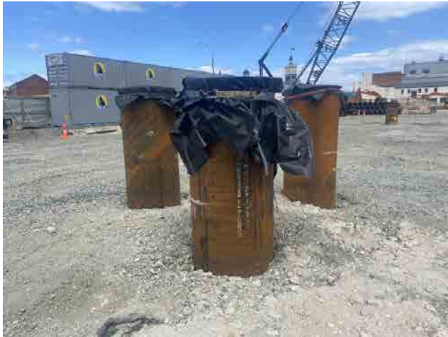
Inpatients Building, a triple pile cluster installed
