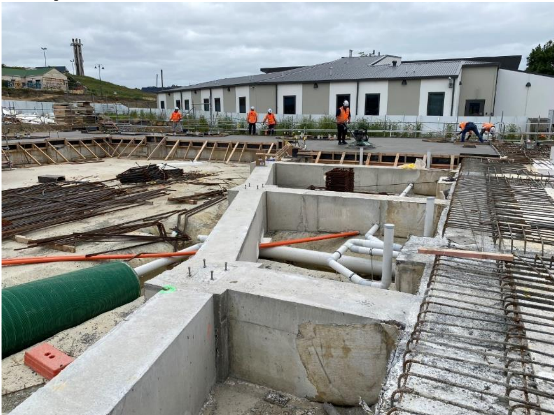
Zone 2 ground beams
